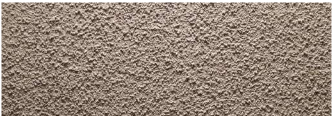
Painted stucco with float sand finish
