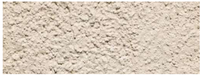
Painted sprayed textured stucco with knocked down finish
